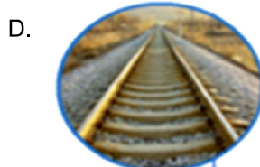
铁轨下面铺放枕木
